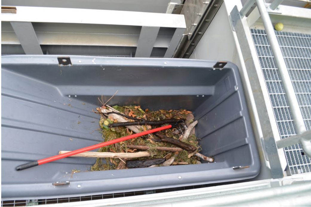
Figure 4-16 - Type of Debris Removed at the North Fork FSC Coarse Debris Rack
